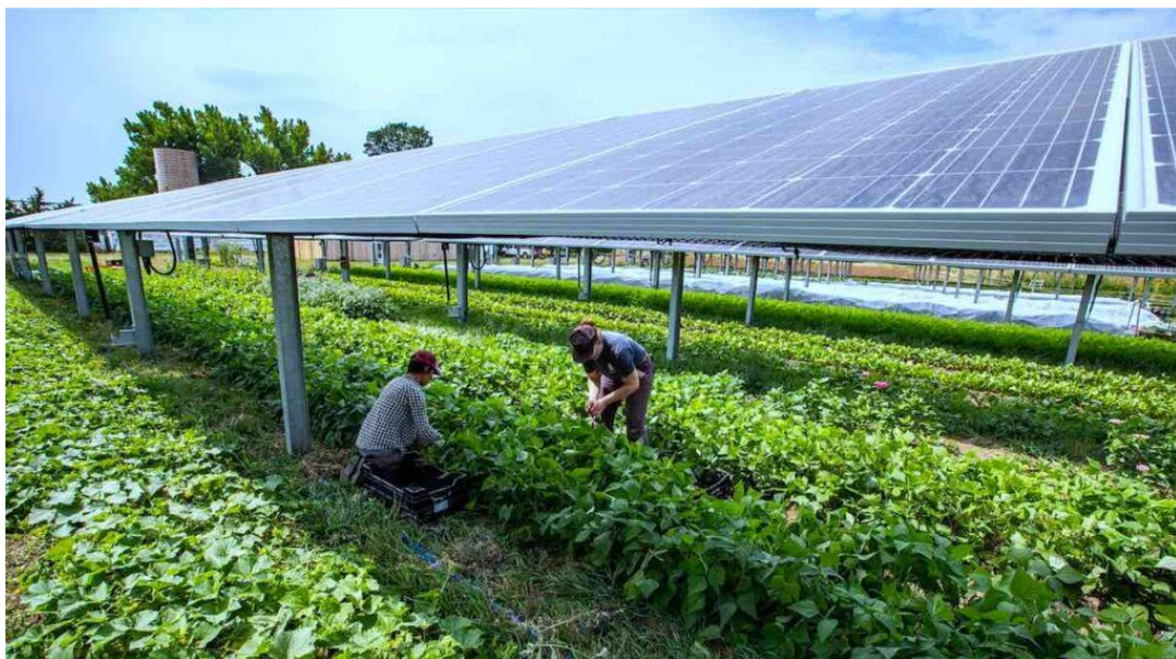
Figure 14. Jack's Solar Farm – Photo by Werner Slocum: NREL
