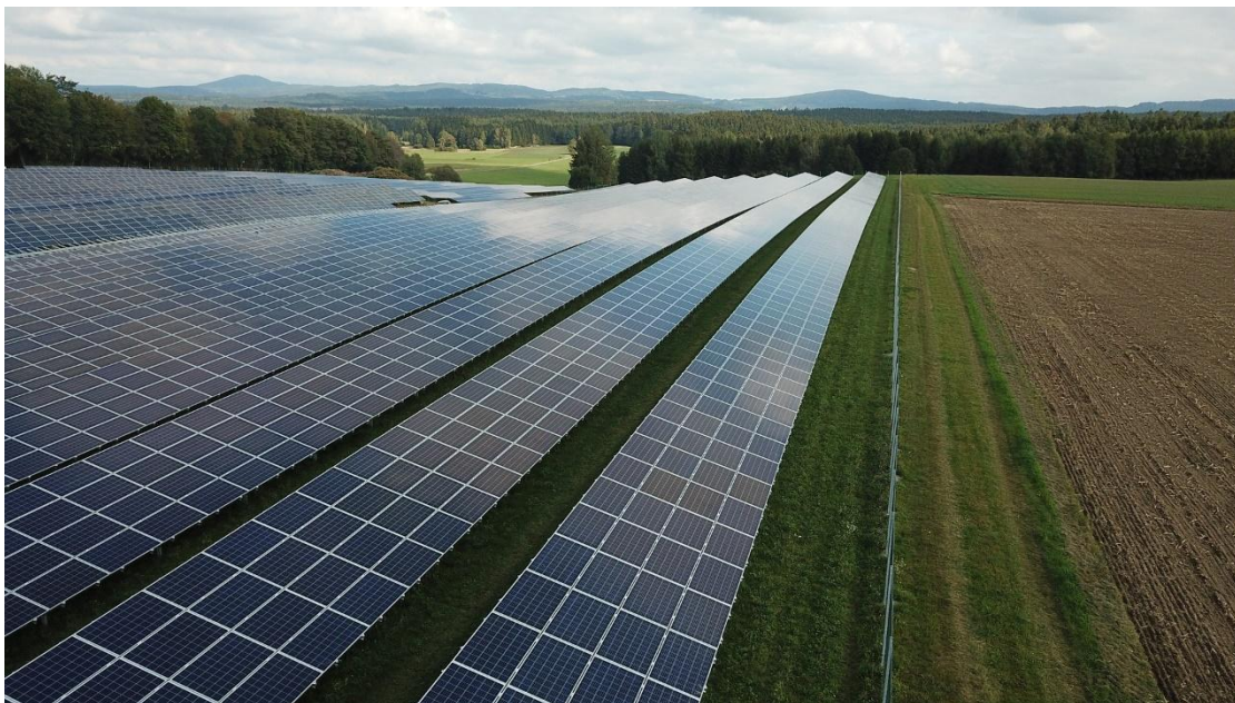
Figura 11 - Photovoltaic Panels - Free picture
