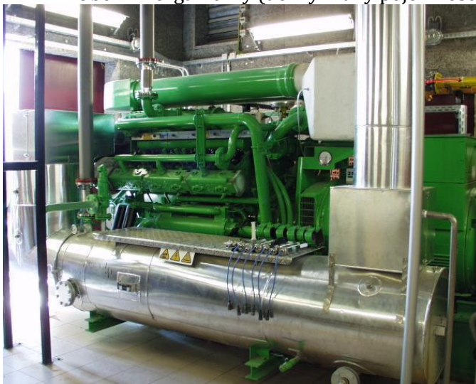
Figure 10 Biogas engine
