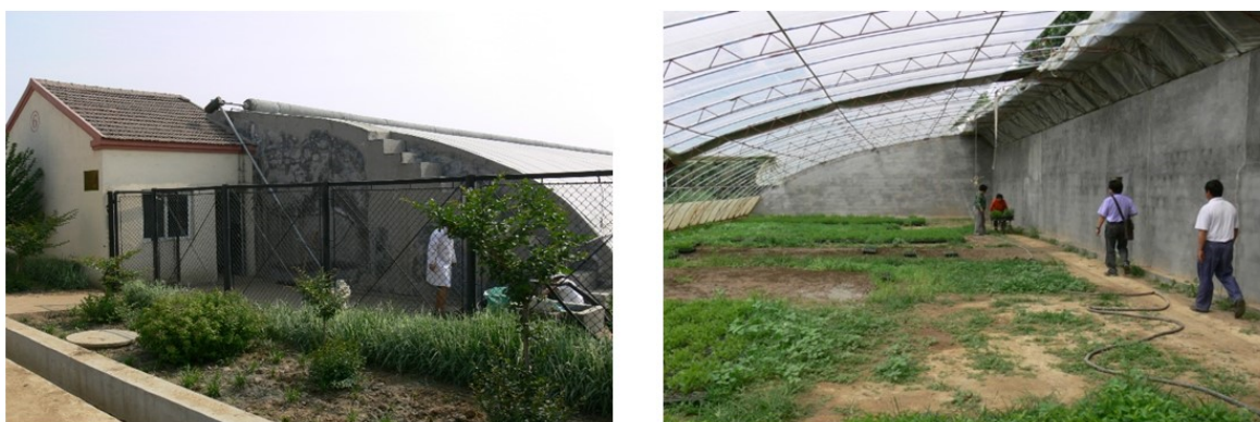
Figure 5 The mat is rolled up at the top of the foil tent
